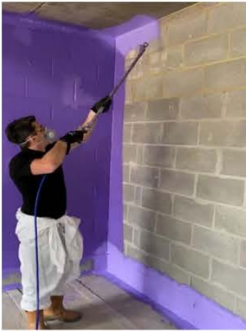
Passive Purple spray install.
