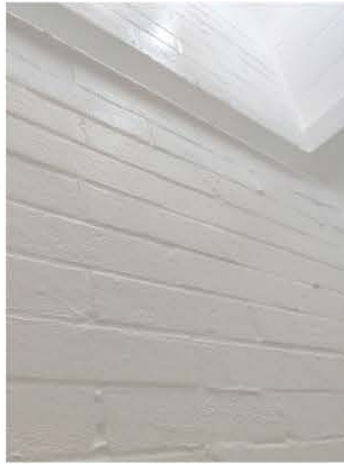
Passive Purple Airtight White Edition retrofit.
