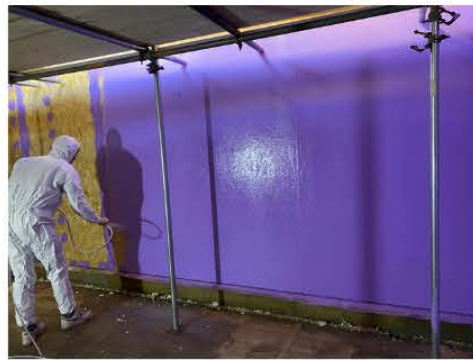
Timber frame wall.
