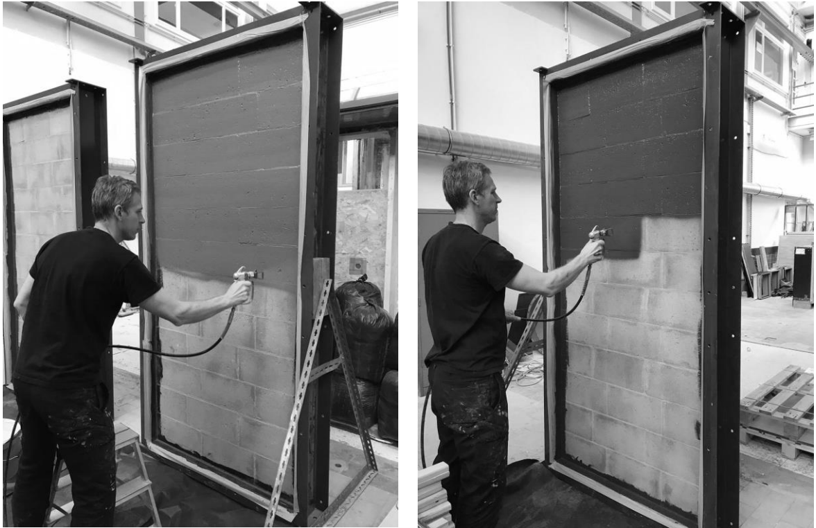
Figures 2: Airless application of PASSIVE PURPLE (left) and PASSIVE PURPLE EXTERNAL (right)
