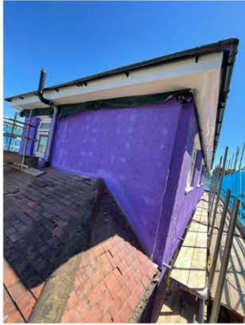
Preparation work on a retrofit.
