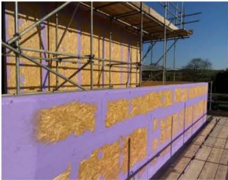
Board joints prepped for application of Passive Purple External.
