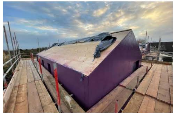
Timber frame install.
