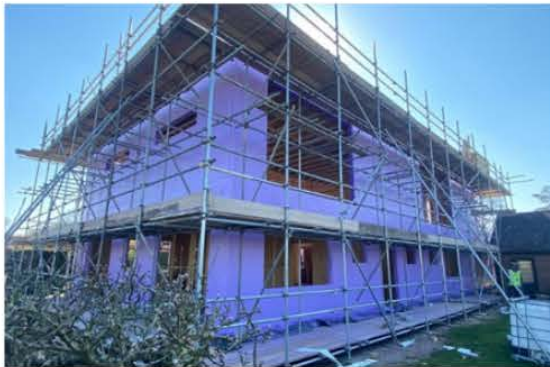
Timber frame install.
