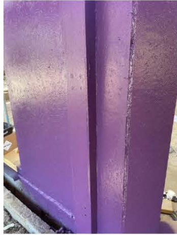
Timber frame install.
