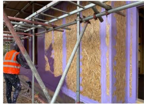
Timber frame wall prepped with Passive Purple External Brush.
