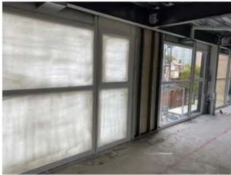
Intelligent Protect install.
