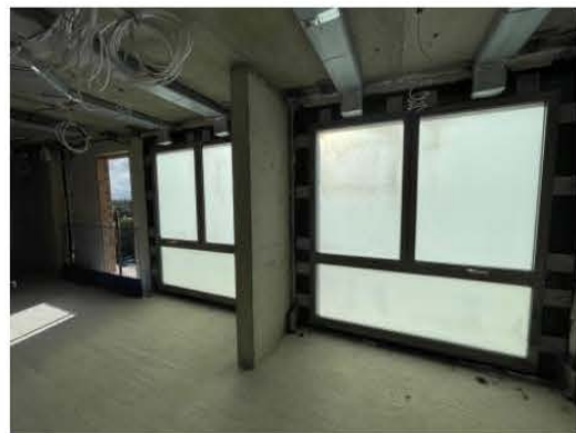
Full temporary protection.
