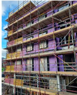
Tower block install.
