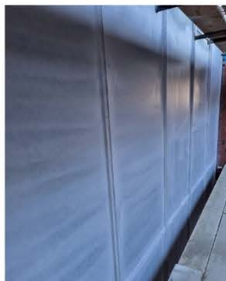
Intelligent Protect install.
