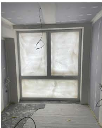
Intelligent Protect install.
