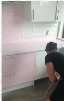
Spray directly on to surface using an airless spray machine.
