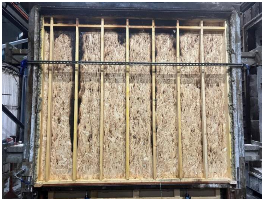
Figure 24 Unexposed face of the specimen after the test
