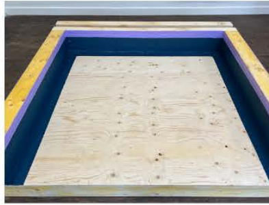
Timber frame, kicker block and sole plate.
