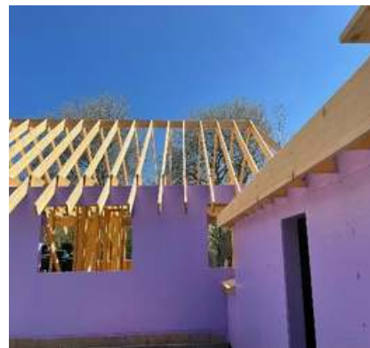
Timber frame install
