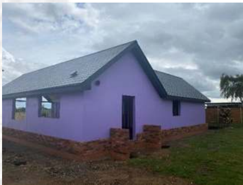
Timber frame install
