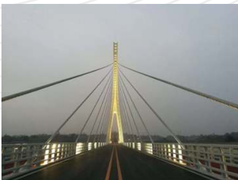
5.3.1 External masonry work on bridge
