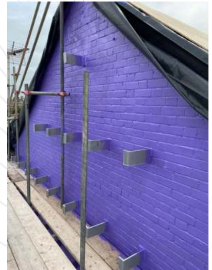
5.1.4 Retrofit- Passive Purple installed insulation
