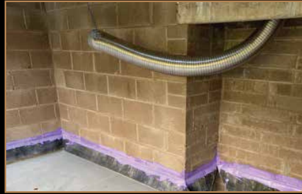
BLOCKWORK TO SLAB/ DPC CONNECTIONS
