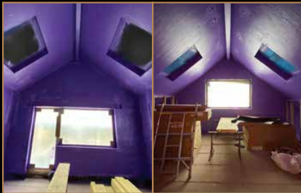
SIPS PANEL ROOF, CAMBRIDGE
