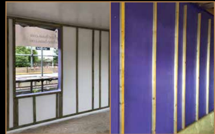
MGO BOARD, PECKHAM (Airtight white and Passive Purple)
