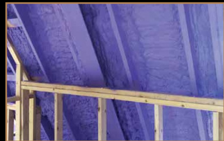
SPRAY INSULATED ROOF, TOTTENHAM
