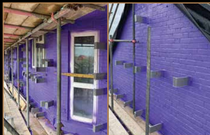
RETROFIT, BEATTIE PASSIVE, GT YARMOUTH
