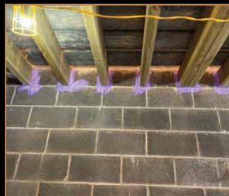
JOIST ZONES INTO BLOCKWORK
