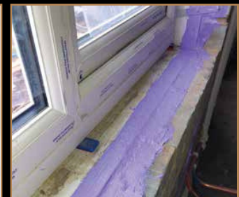
WINDOW/DOOR UPVC FORMERS TO BLOCKWORK
