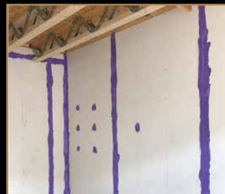
MGO BOARD JOINTS AND FIXING PENETRATIONS
